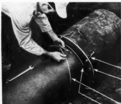
Assembling cable with rubber-covered union for clamping gasket lip to pipe.
